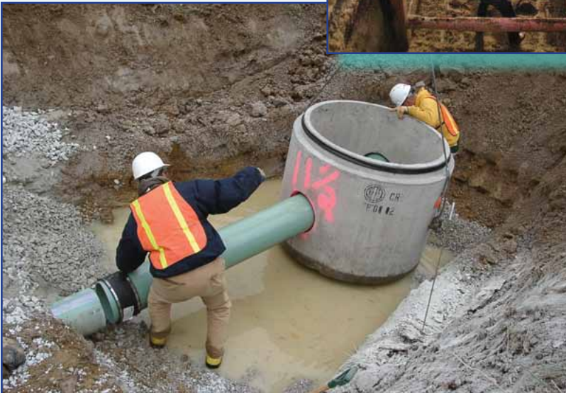
Storm sewer construction underway.
